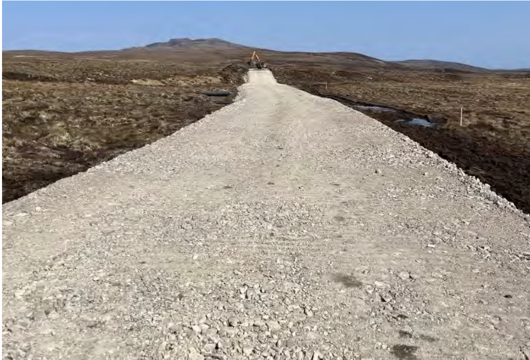
Figure 2-12: Floating Road Embankment
